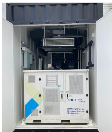
CLPe designs a compact and lightweight Battery Energy Storage System (BESS) especially for mobile and small-scale power applications, which is about 20% of the size and weight of a standard BESS. This helps reduce carbon emissions by replacing the use of conventional diesel generators.
