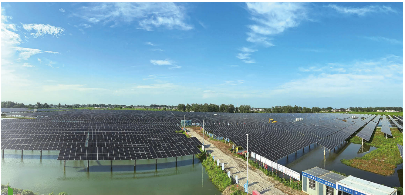
The new Yangzhou Gongdao Solar Power Station in Jiangsu province is equipped with an 8MW commercial use battery energy storage system, the first of its kind in the province.
