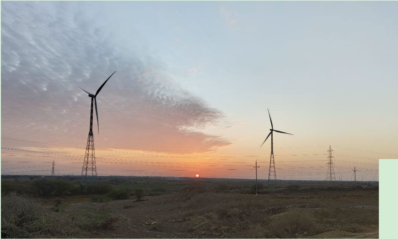
Sidhpur wind farm located in the state of Gujarat, India.
