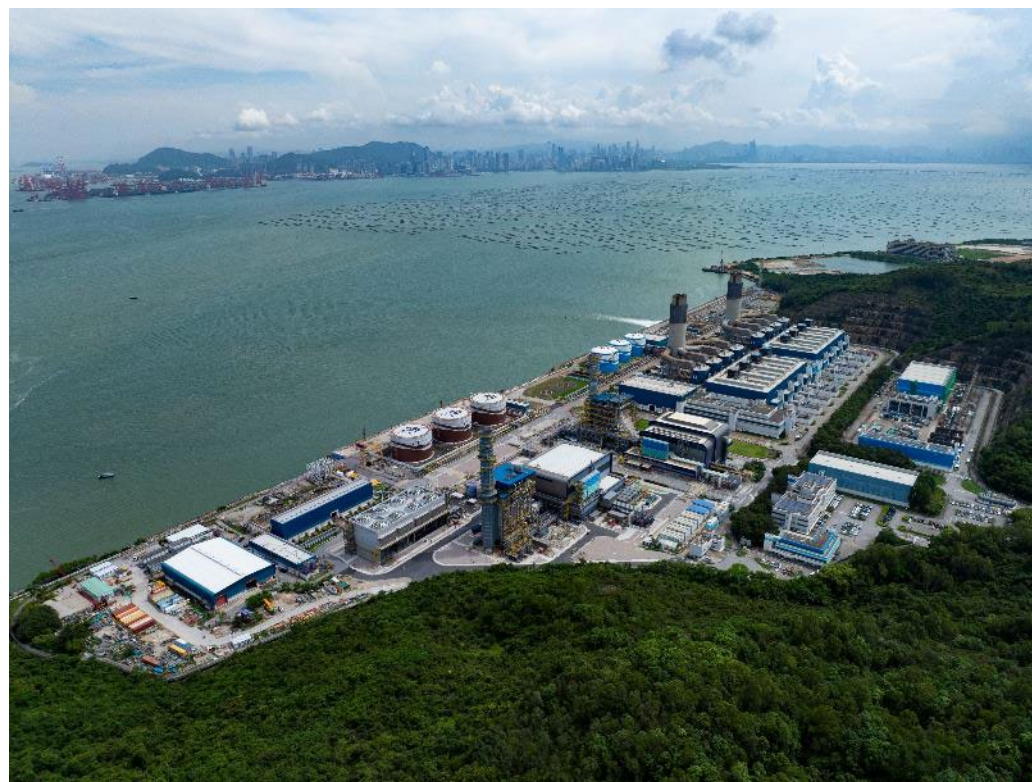
Black Point Power Station in Tuen Mun, Hong Kong.
