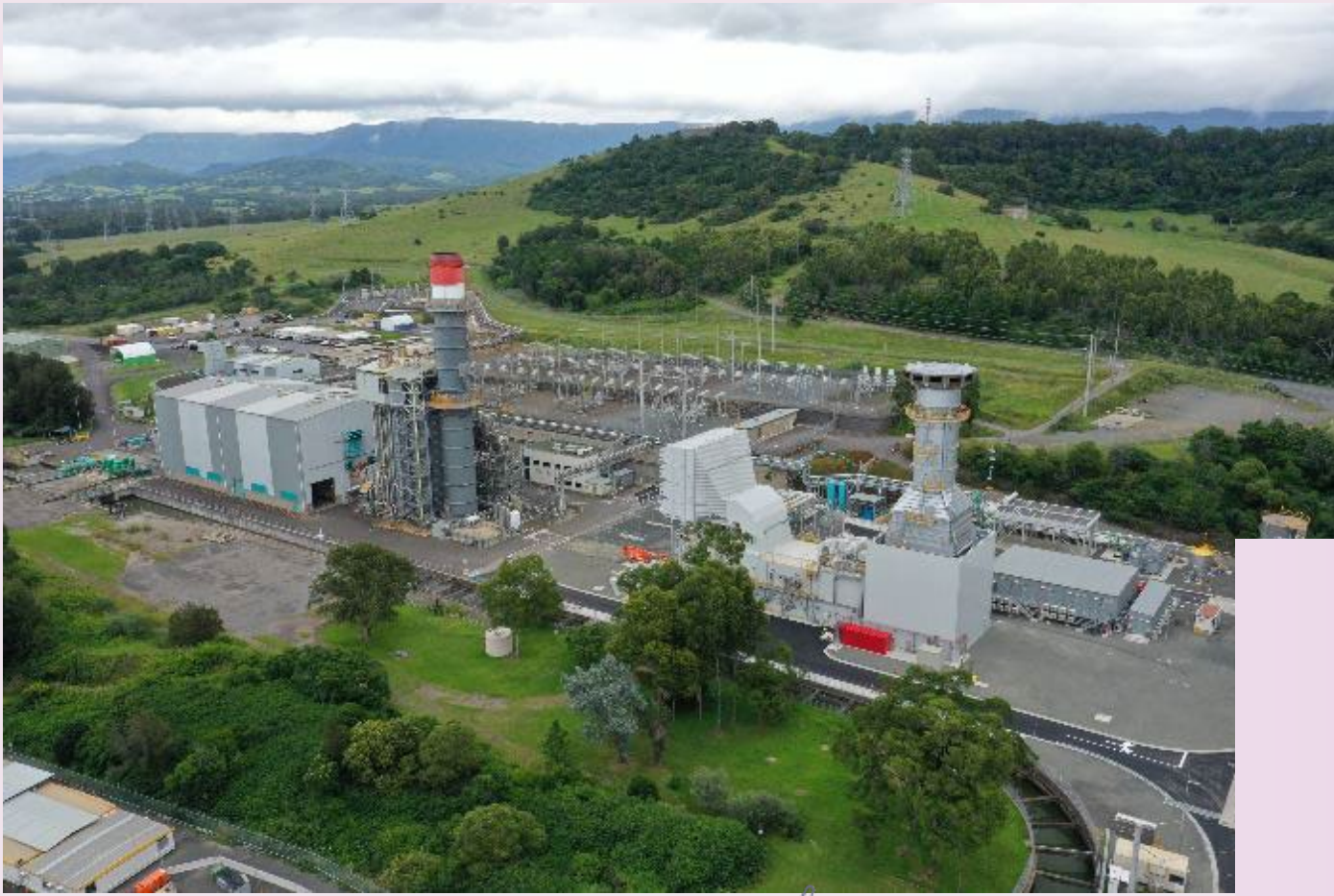
Tallawarra gas-fired power stations A & B in New South Wales, Australia.
